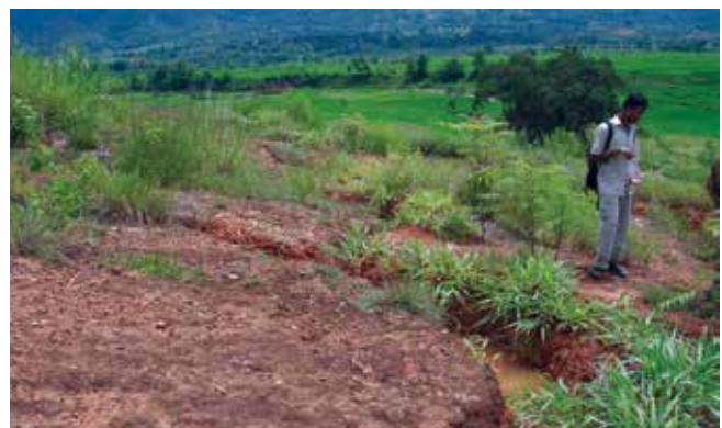
Figure 56: A combination of trenches, eyebrow pits and tree plantation to harvest surface runoff and increase infiltration
