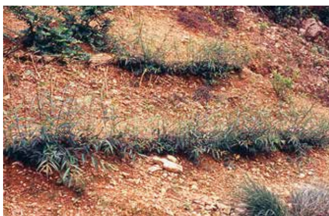
Figure 53: Brush layering across slopes along a contour
