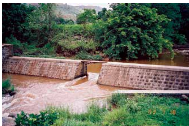
Figure 30: Discharge measurement using rectangular weir arrangement and measuring the head in the weir
