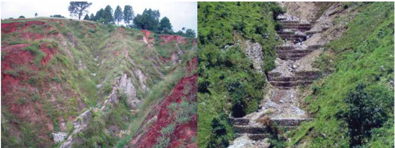
Figure 50: Check dams constructed along gullies to control erosion and increase infiltration
