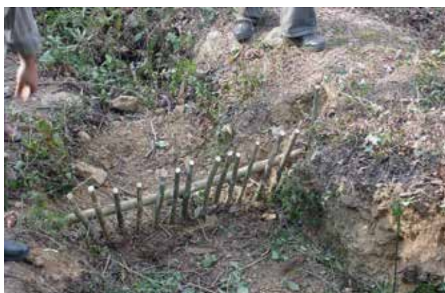
Figure 53: Brush layering across slopes along a contour
